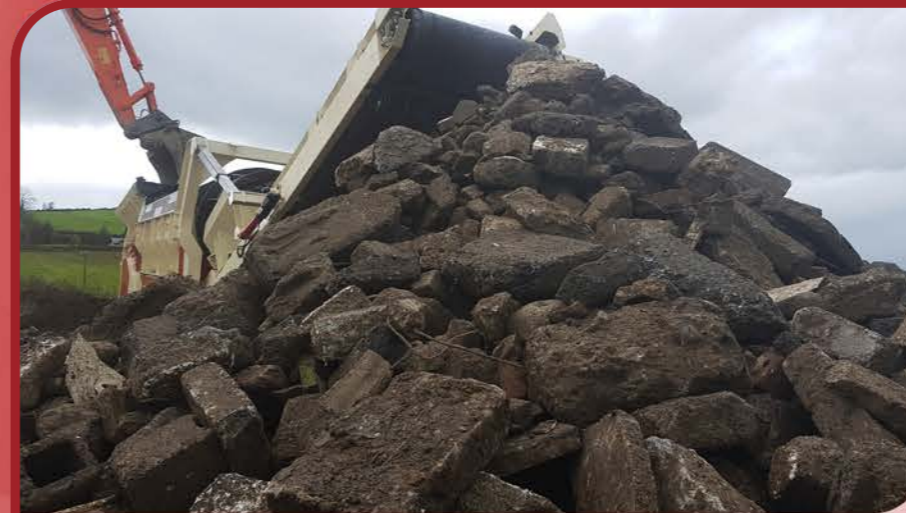
Concrete and bricks removed from the demolition waste
