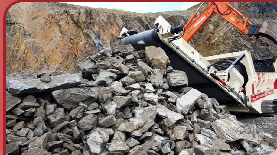
Clean blasted rock from Oversize
